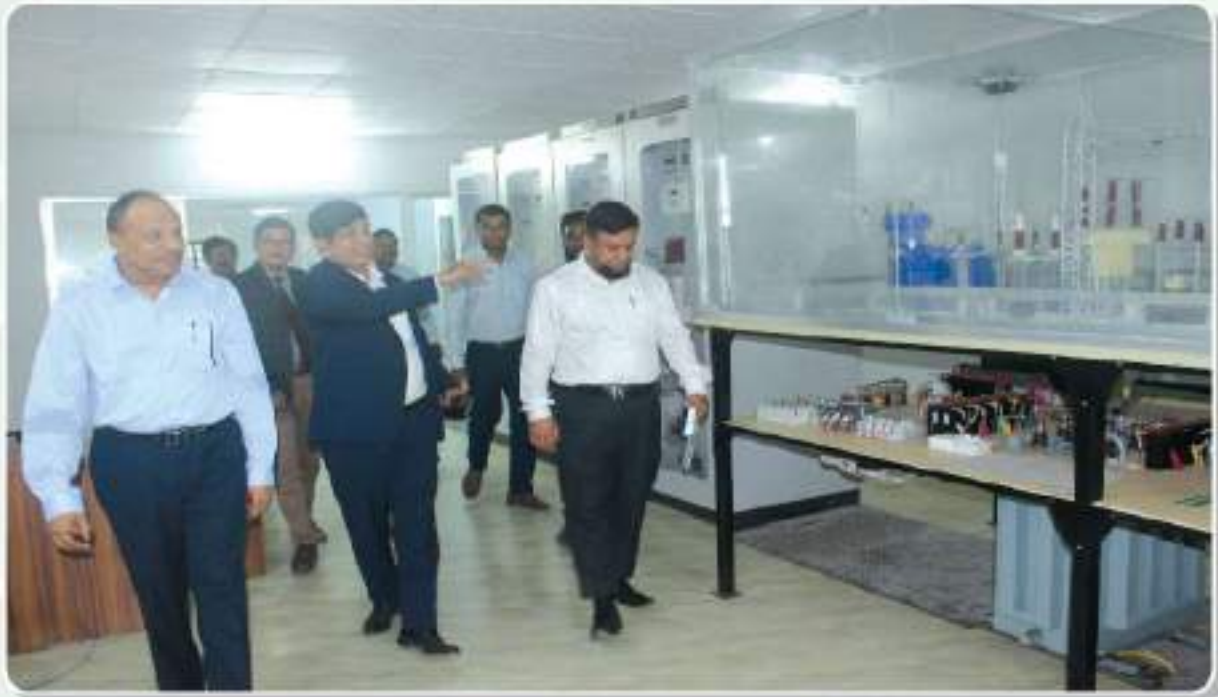
Honourable Chairman, WZPDCL visiting newly constructed Model Sub-Station.
