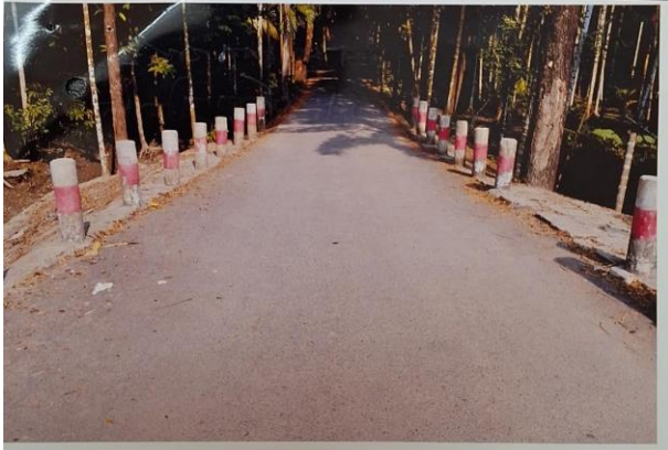
Construction of 16.00m Long RCC Girder Bridge on Maniram Munshir hat to Tabgi Road at Ch.13m. ID No. 509215113 under Borhanuddin Upazila, District- Bhola
